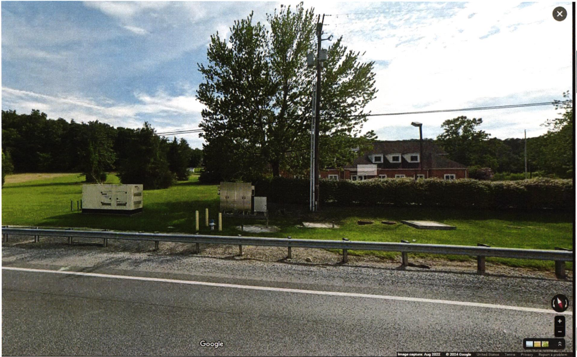
Photo: Western Virginia Water Authority Clearbrook Sanitary Sewer Lift Station US 220 South
